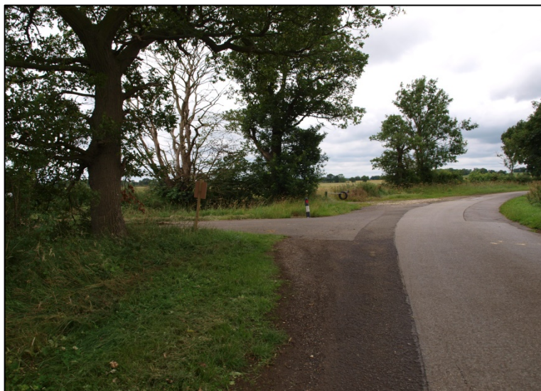
1. Site entrance and access onto Smithfield Road
